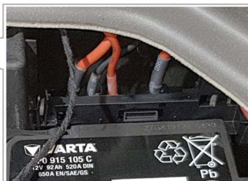
Main fuses (SA) of the battery
